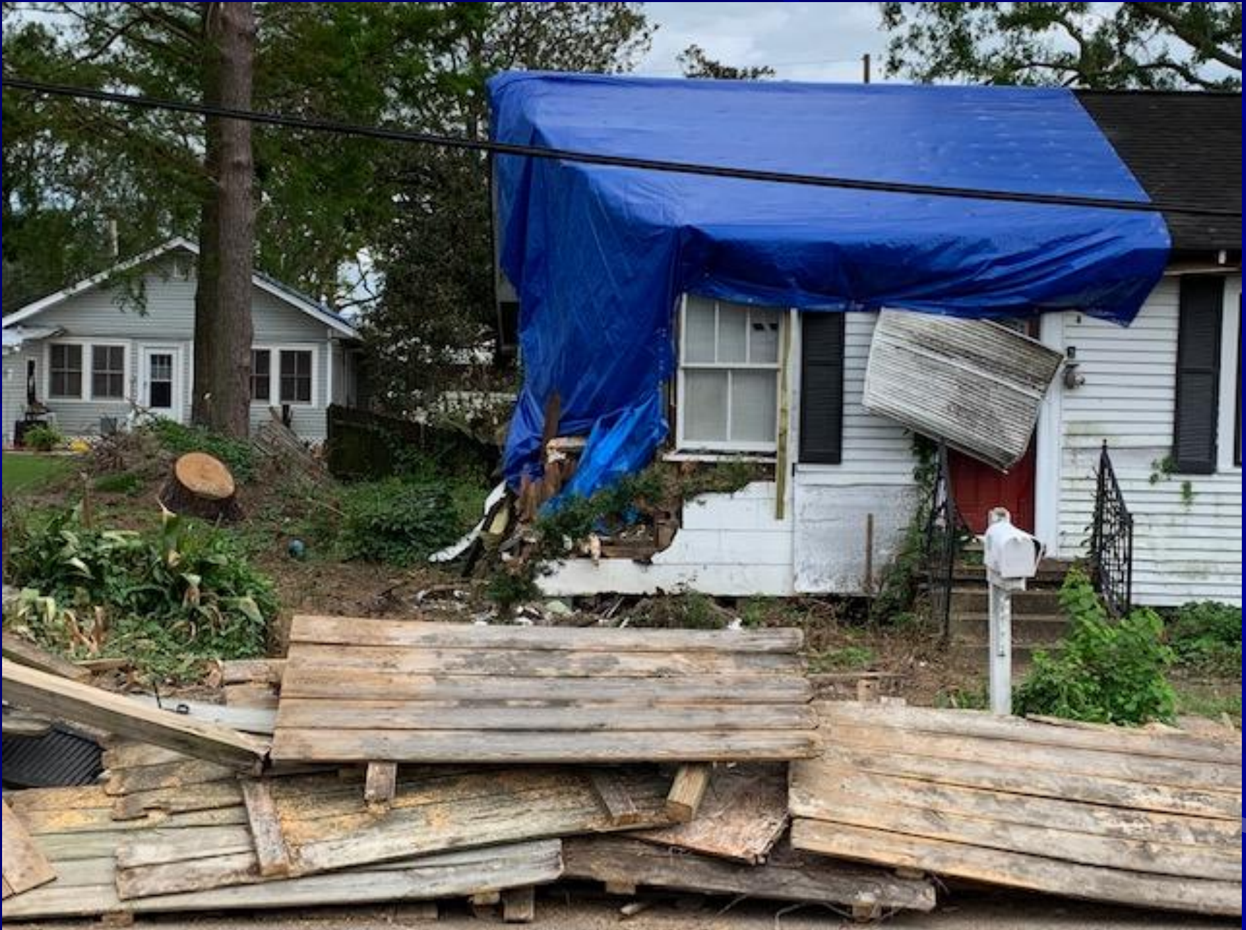
Hurricane Ida damage, NORCO, LA
